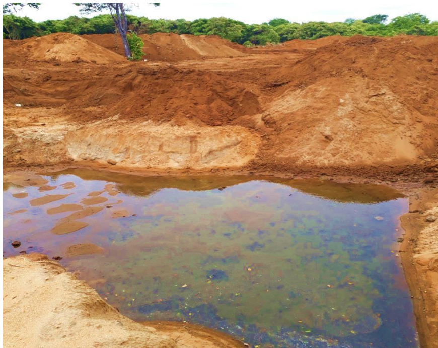
Deep pits in the reservoir premises
