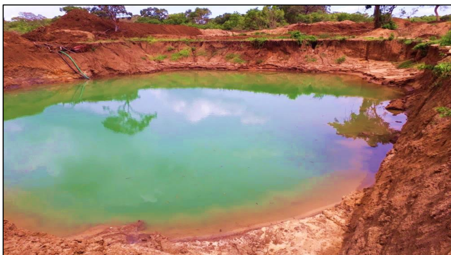
Deep pits in the reservoir premises
