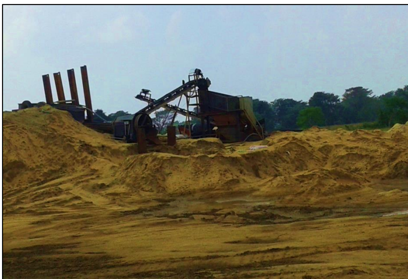
Sand exaction machines
